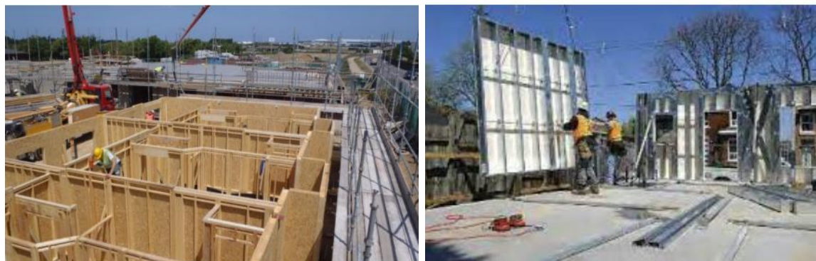
Figure 3 Timber walls [7]. Figure 4 Prefabricated Light Steel Framing [14]
