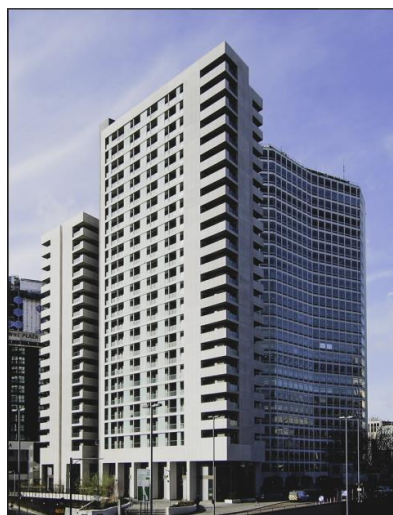
Figure 5 Precast concrete constructions, Arena Central, Birmingham, 2019 [13]
